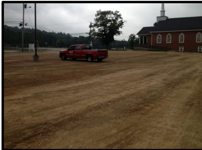
Figure 8 Compacted Fill Lot
